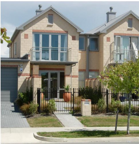
PHOTO 6 - PROVISION OF A CLEAR ENTRANCE AND BALCONY FRONTING THE STREET (NORTHWOOD, CHRISTCHURCH)
