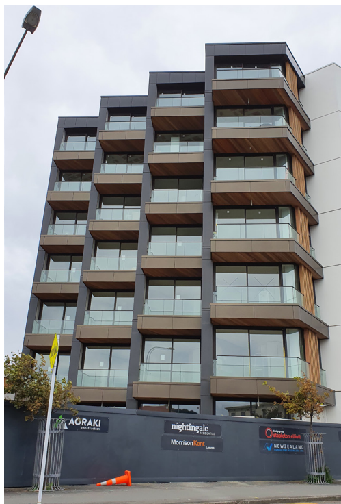
PHOTO 11 - STAGGERED BALCONIES MAXIMISE PRIVACY WHILE RETAINING OUTLOOK AND SUNLIGHT ACCESS (WELLINGTON)
