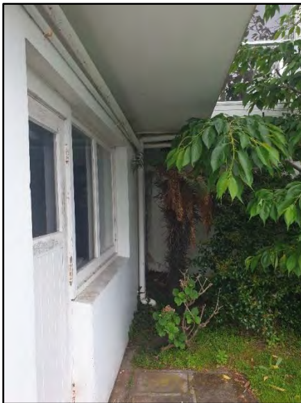
Figure 6 – Downpipe junction on eastern face of dwelling
