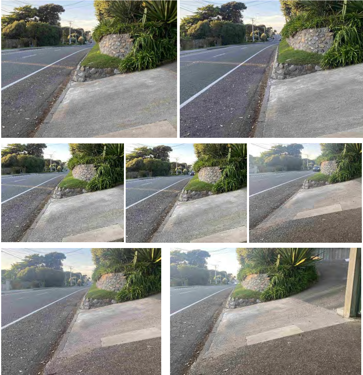
Figure 7: Views north from the House 1 garage driveway
