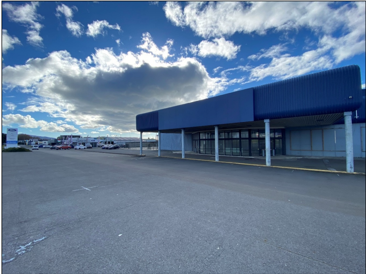
Figure 8: View of the site looking to the north and the building to be demolished
