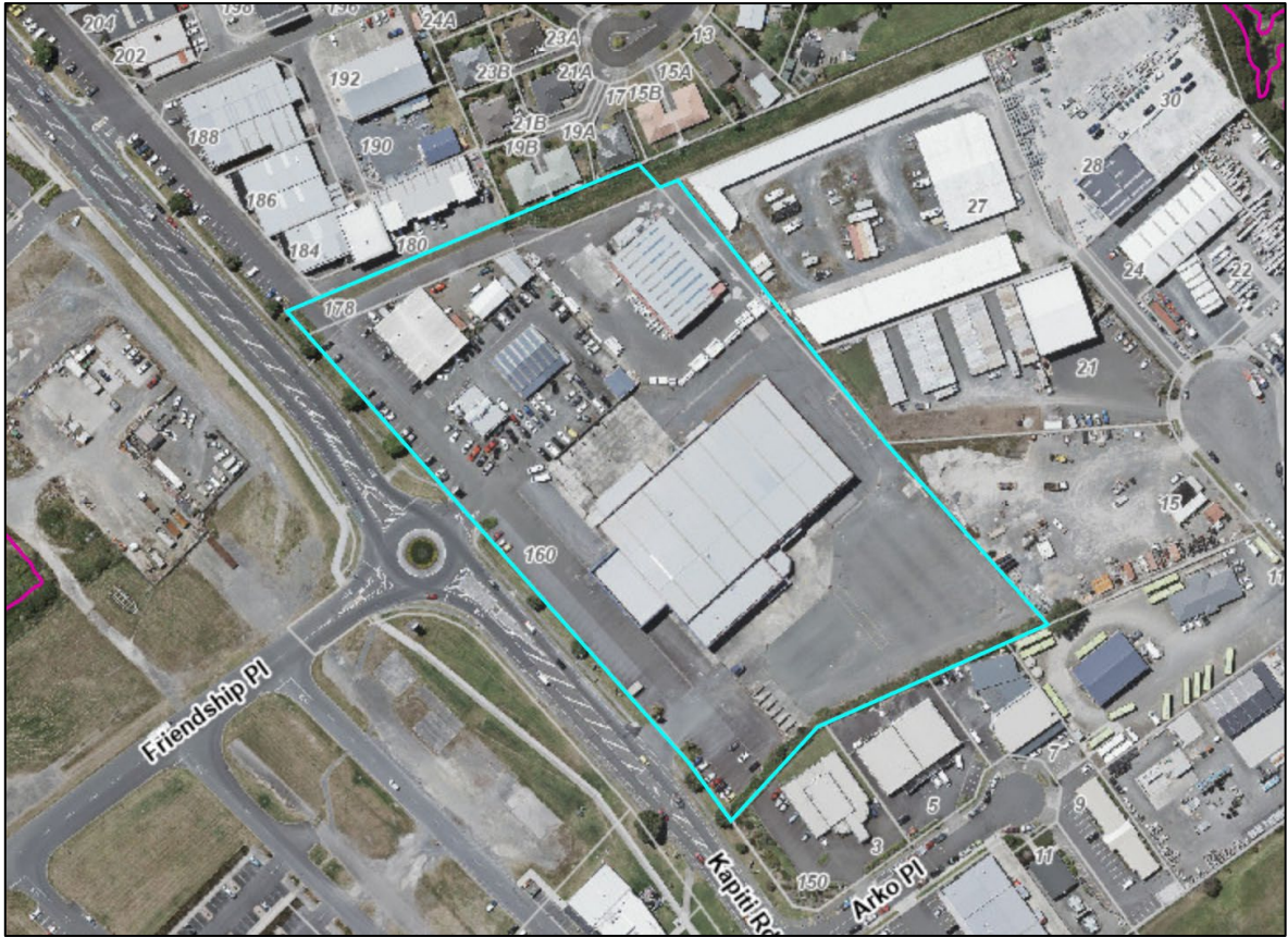
Figure 6: Aerial image of the subject site (bordered in blue) and surrounding environment
