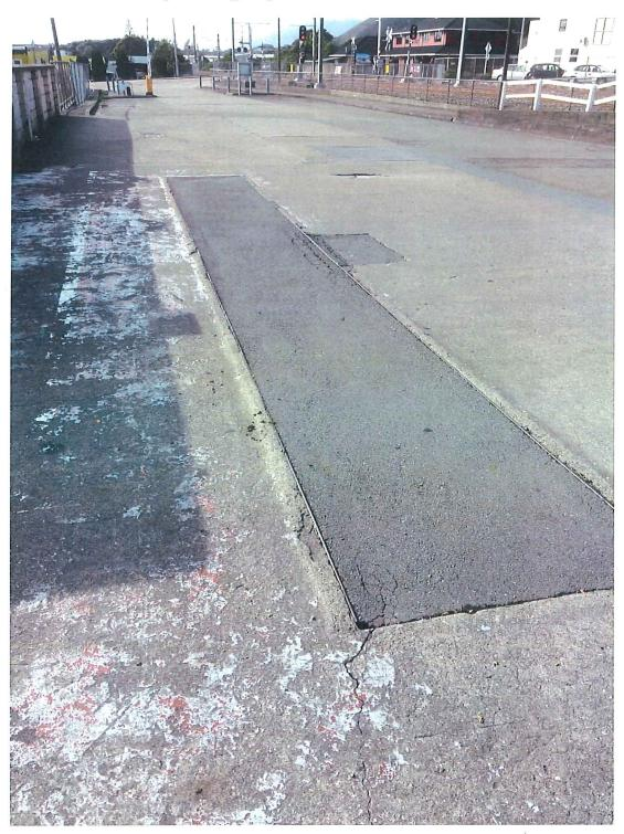
Plate 1. The northern extent of the site, photographed from the centre looking north. In the foreground is the foundation slab of the former workshop, with the infilled bus inspection pit clearly visible. Rectangular patches further away, past the manhole, appear to be the locations of the former USTs. The Kapiti Road entrance is at the top of the image.
