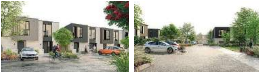
Fig. 2: Exterior views of 240 Kapiti Road
