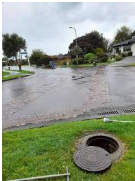
Above: 15 th October 2021 – Existing sewer manhole on Halsey Grove
