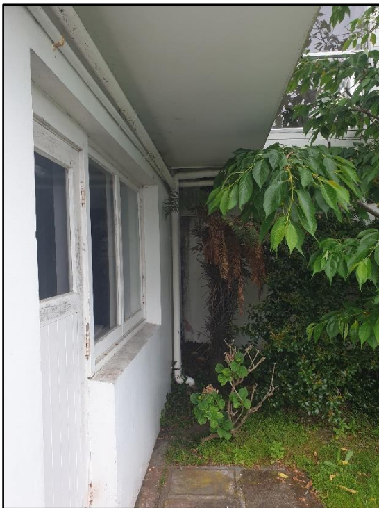
Figure 6 – Downpipe junction on eastern face of dwelling
