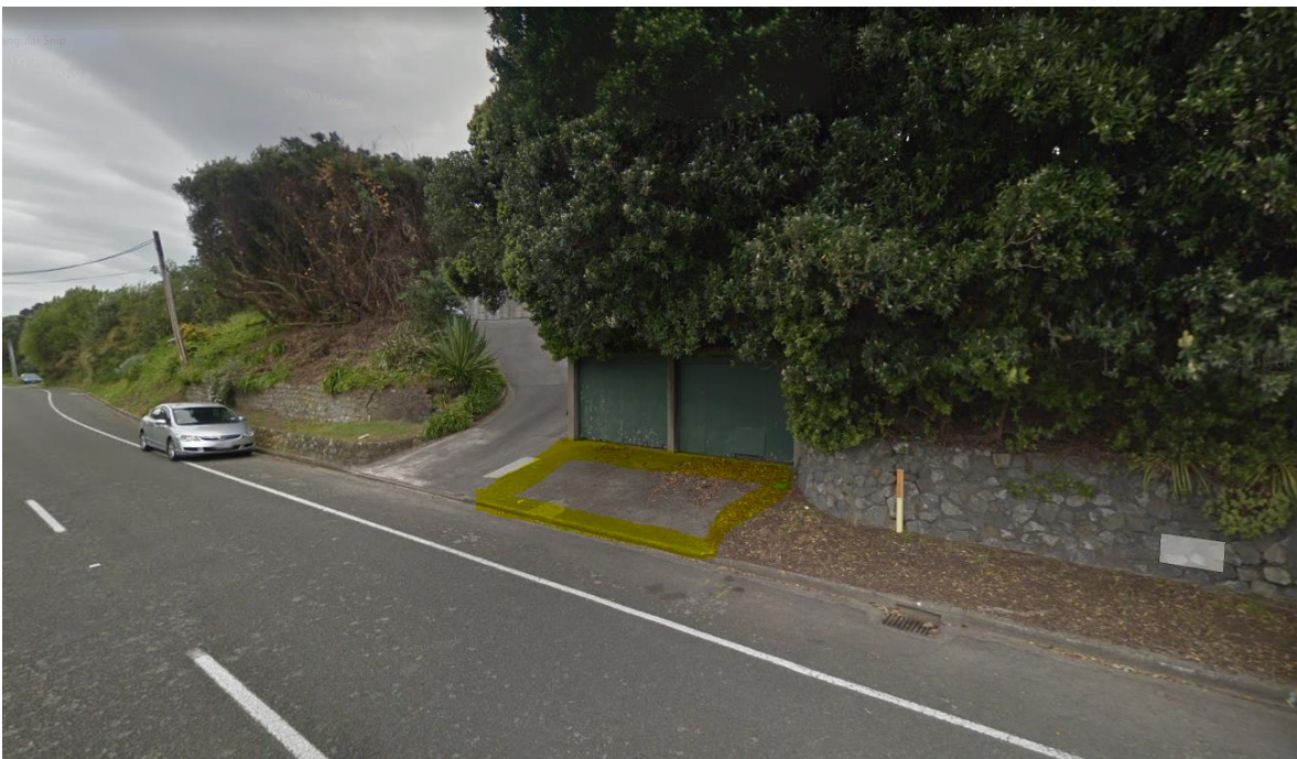
Figure 2 - Northern crossing off Rosetta Road used for basement garage
