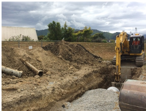
Stormwater upgrade at Charnwood Grove - Phase 1
