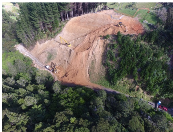
Waterfall Road earthworks underway
