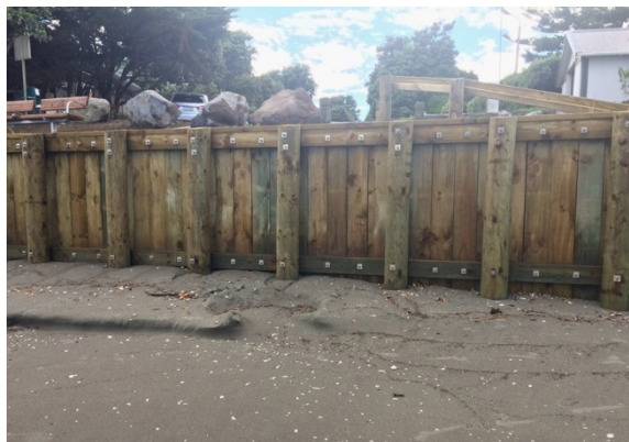
Arawa Street replacement seawall
