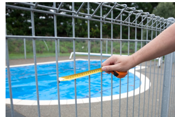
Inspecting pool fencing compliance
