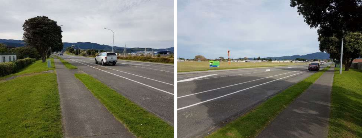
Figure 3: View east (left) and west (right) along Kapiti Road
