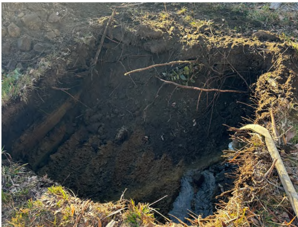
Above: 8 July 2024 – Underlying sand material in test pit
