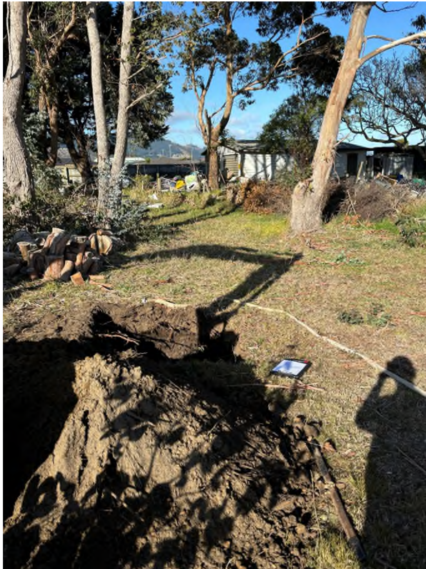
Above: 8 July 2024 – Looking south with test pit shown
