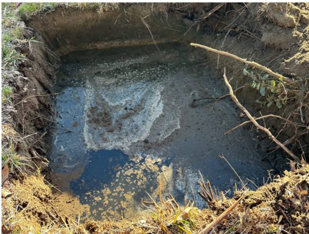
Above: 8 July 2024 – Test pit during testing
