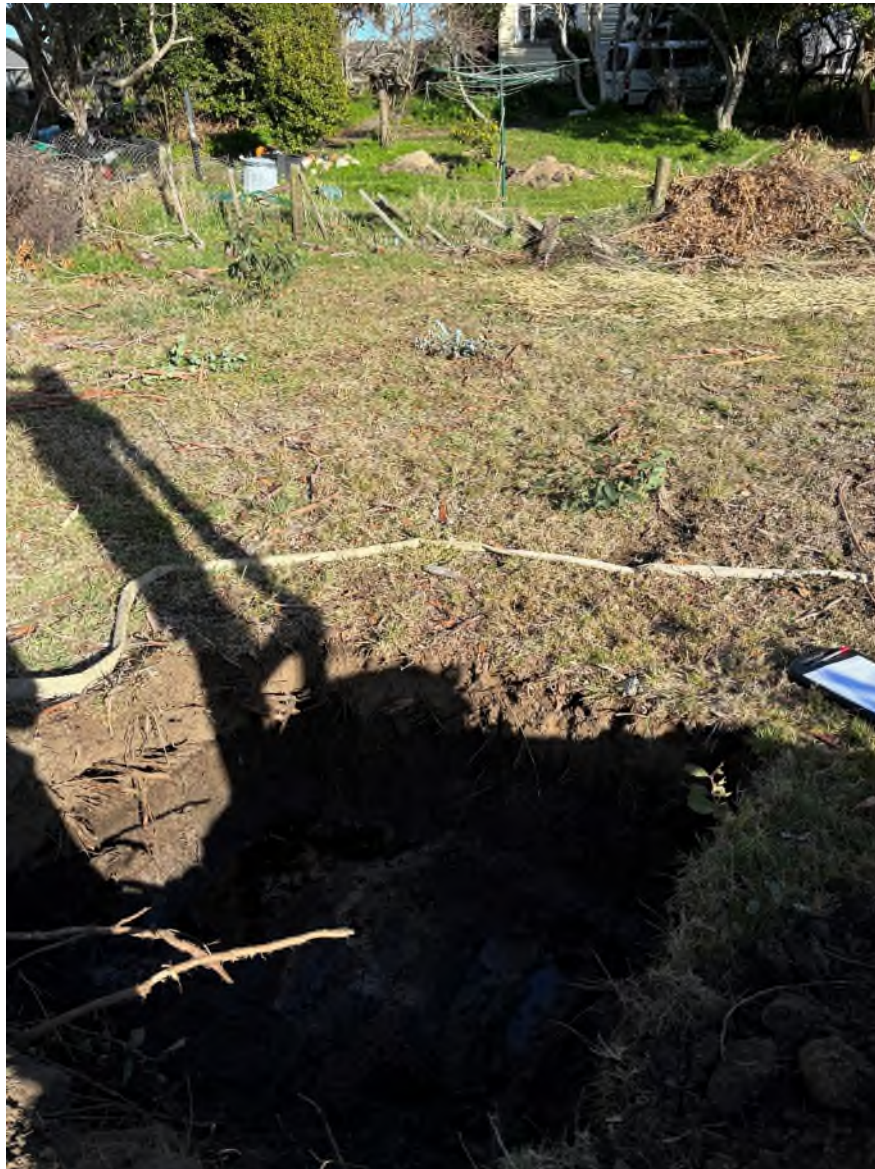
Above: 8 July 2024 – Looking southwest with test pit shown
