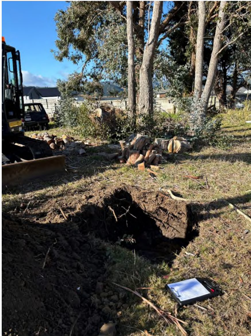
Above: 8 July 2024 – Looking southeast with test pit shown
