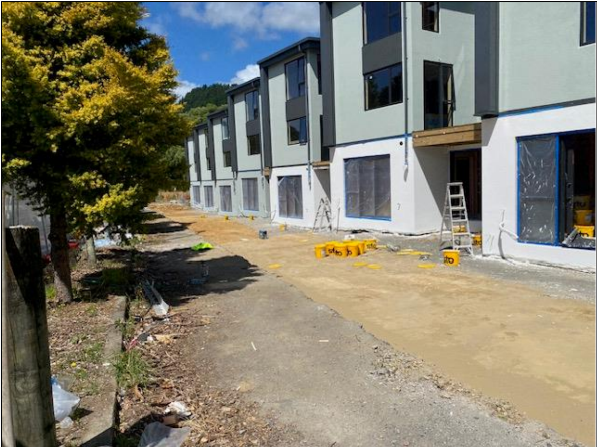
Figure 6: View of the northern townhouses, Principal Units 2, 4, 6, 8, 10, 12 and 14)
