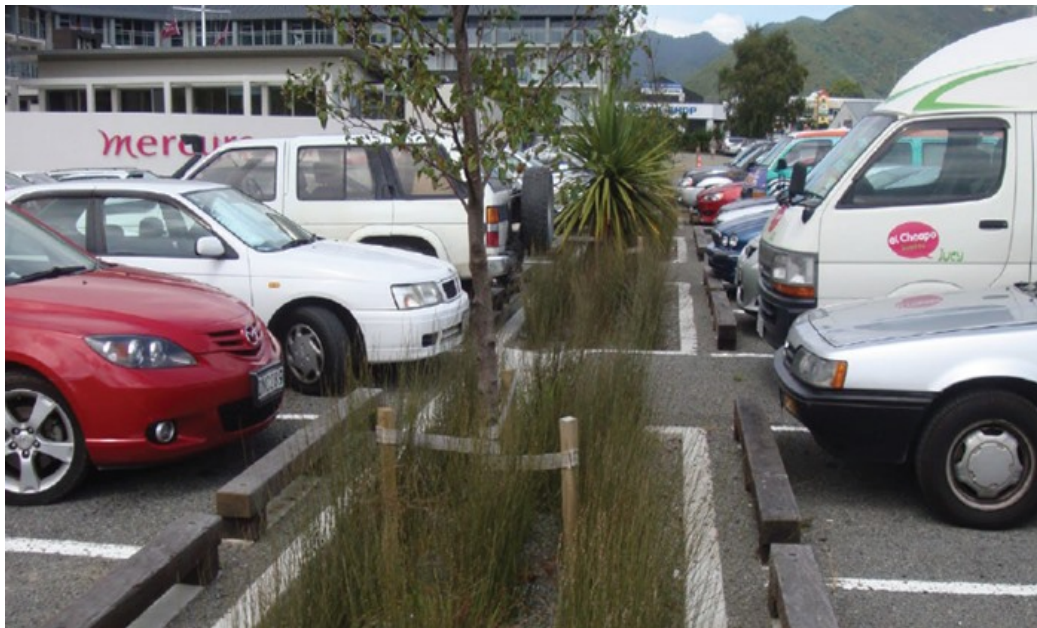
Photo 3 - Landscape treatment and rain gardens as part of parking lot
