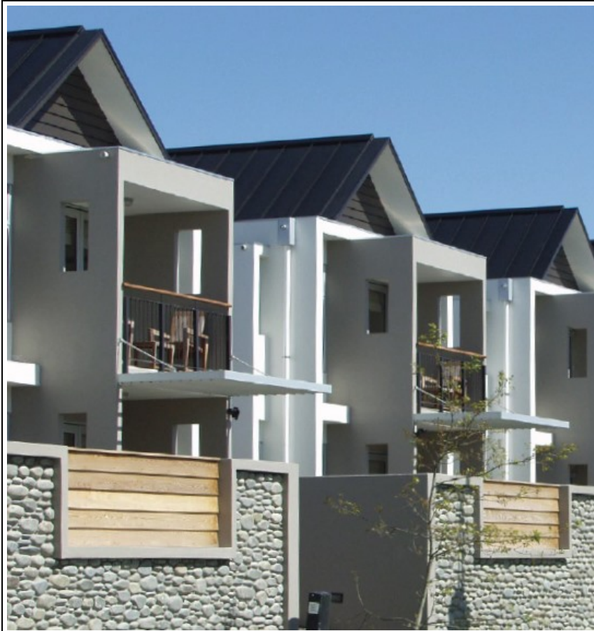
Photo 10 - Overhanging balconies provide shade in summer (Clearwater Gold Resort, Christchurch)
