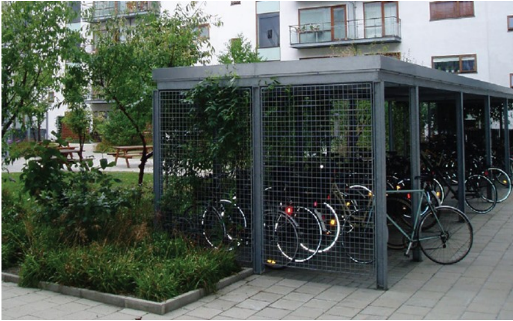
Photo 1 - Sheltered and screened bicycle parking
