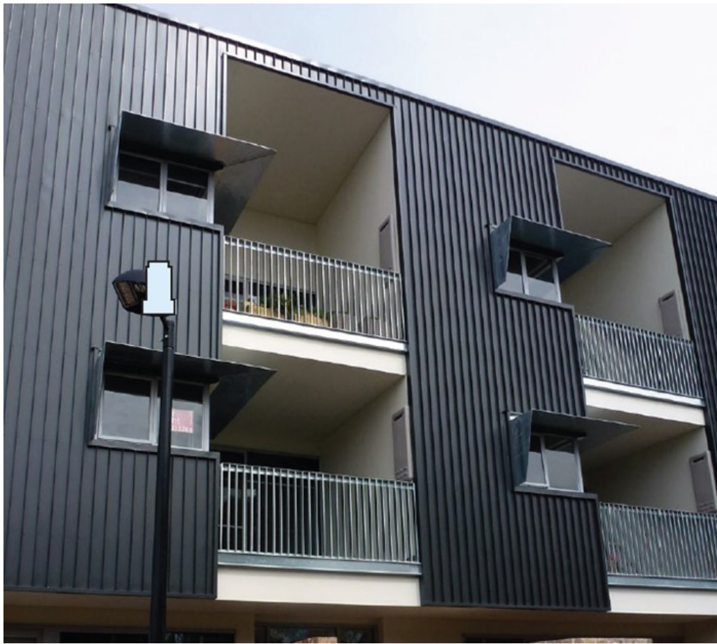
Photo 4 - Strategically integrating balconies into the design can enhance the sense of privacy
