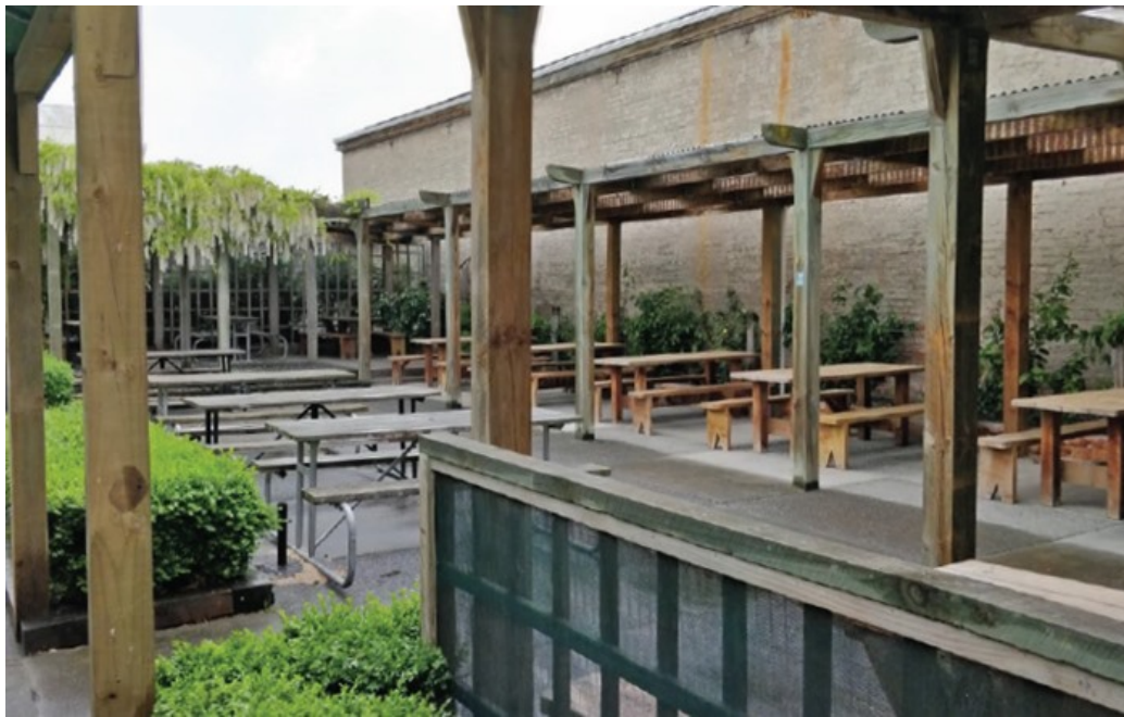
Photo 5 - Court yards away from vehicle routes can create comfortable intimate and sheltered spaces, Martinborough
