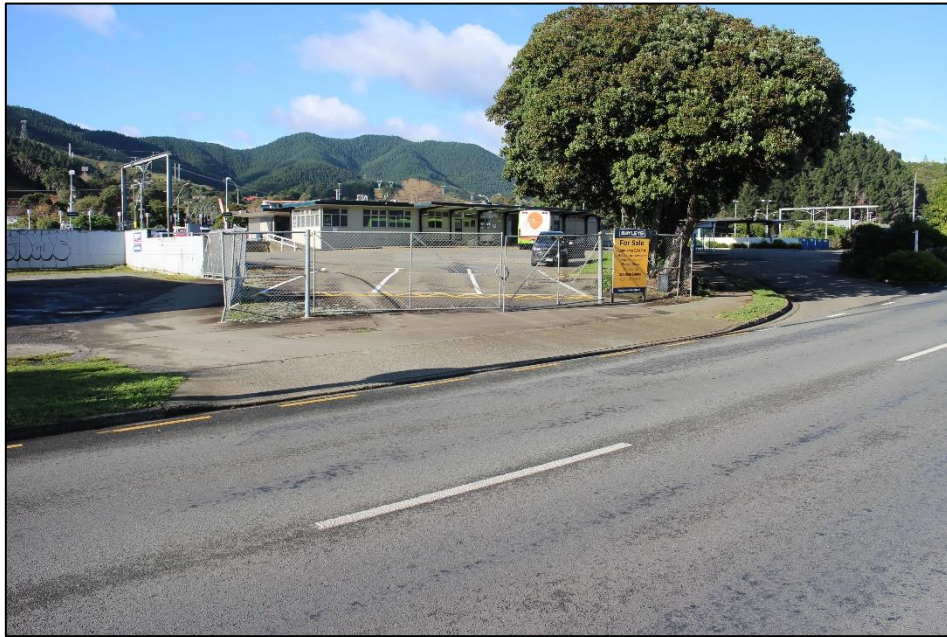
Photograph 1: The Site, Viewed From Amohia Street.
