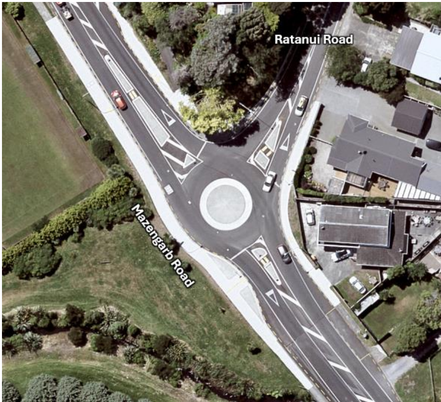
Figure 3-1: Mazengarb Road / Ratanui Road Intersection (Aerial Image Source: Emap)
