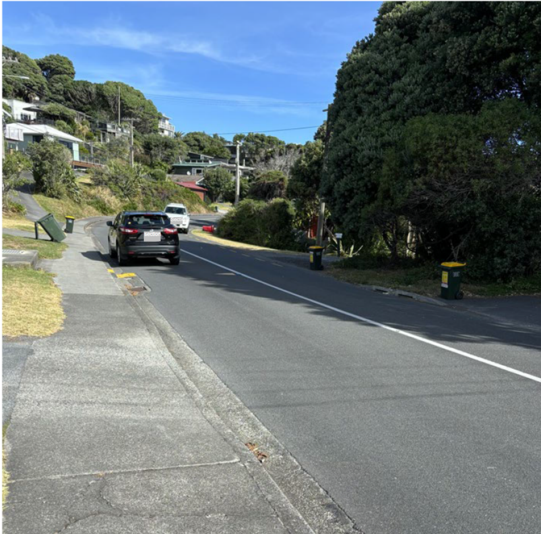
Figure 2: Looking south along The Esplanade
