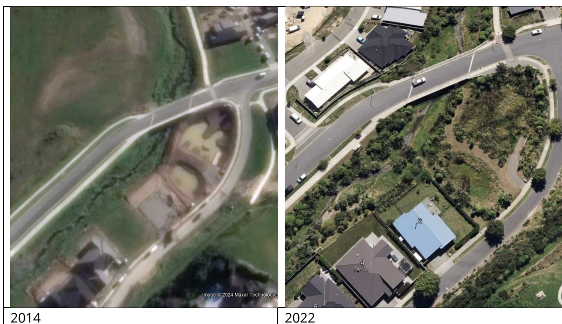
Figure 6. Todd Upper Duck Creek stormwater conversion post construction to wetland.
