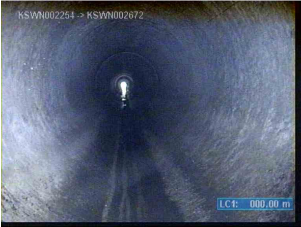
KSWP004512_78f79a2c-7a30-477a-bdf6-03125de5751b_20220711_125340_084.jpg, 00:00:12, 0.00m Inspection start, node reference: KSWN002254
