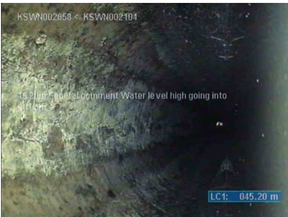
KSWP004528_519b205c-9559-4adf-97c9-13e5ab0f0c8c_20220809_112722_172.jpg, 00:08:11, 45.20m (3.50m) General comment / Water level high going into stream
