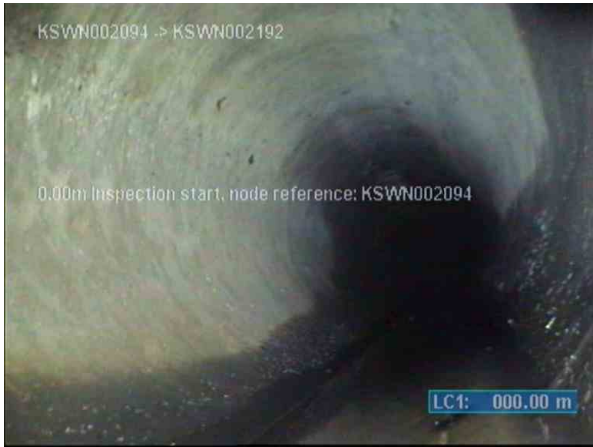
KSWP003817_224e464b-ab95-4ae6-aa2d-987a188d07f9_20220812_112800_348.jpg, 00:00:17, 0.00m (56.00m) Inspection start, node reference: KSWN002094
