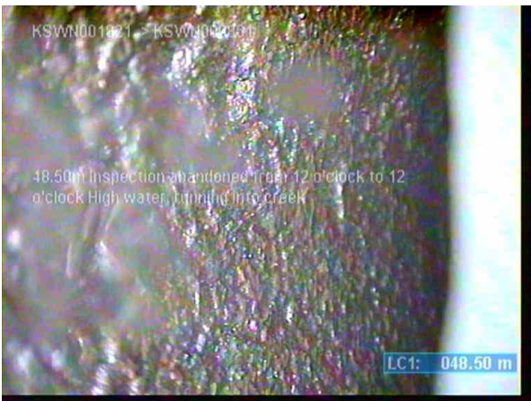
KSWP003815_c7aa7907-fc96-4a78-b240-7bb6f4c7ad22_20220701_140011_875.jpg, 00:11:27, 48.50m Inspection abandoned from 12 o'clock to 12 o'clock / High water, running into creek
