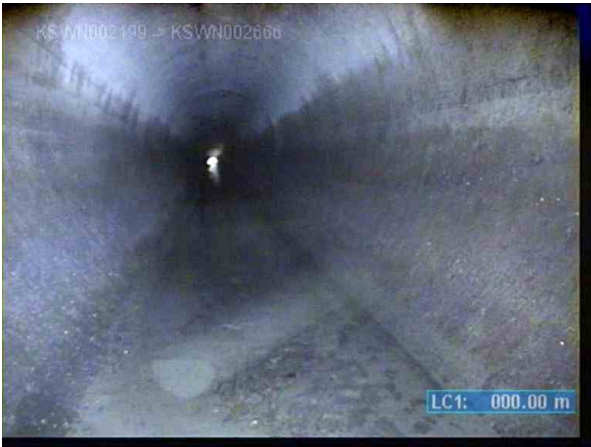
KSWP003760_7677c142-fac2-4d80-89f4-e9575e26f6a4_20220729_130055_240.jpg, 00:00:12, 0.00m (55.40m) Inspection start, node reference: KSWN002199
