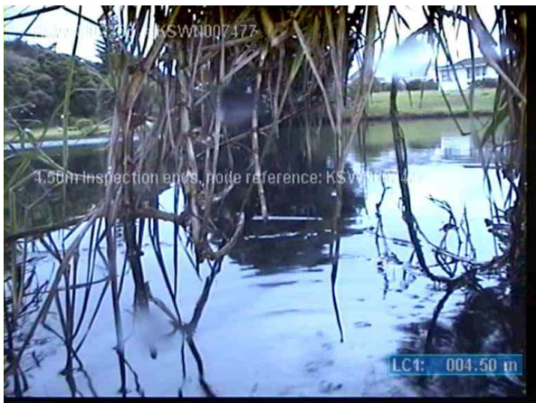
KSWP003634_e8054480-66f1-423c-82c9-a92725071798_20220708_155606_909.jpg, 00:02:28, 4.50m Inspection ends, node reference: KSWN007477
