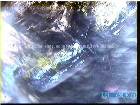
KSWP003760_8a078897-305d-4a67-b1bc-06dc3754d98b_20220729_130517_633.jpg, 00:04:25, 55.40m (0.00m) Inspection ends, node reference: KSWN002666
