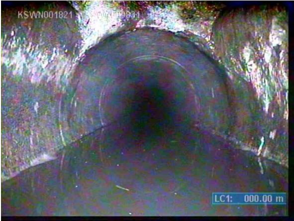
KSWP003815_55591706-00c2-44c2-bdff-3145507a1a94_20220701_134803_749.jpg, 00:00:10, 0.00m Inspection start, node reference: KSWN001821
