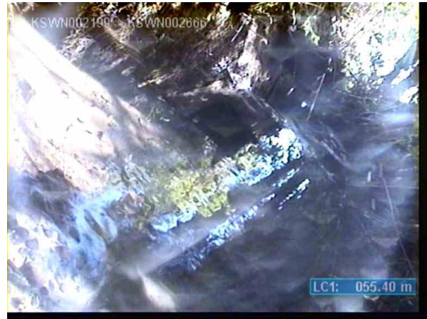
KSWP003760_eb9b8076-ced0-4af8-a24e-2047390a5156_20220729_130513_621.jpg, 00:04:25, 55.40m (0.00m) Inspection ends, node reference: KSWN002666
