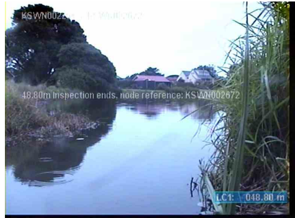
KSWP004512_087bebea-fdb2-4655-9c99-90565d25f838_20220711_125923_108.jpg, 00:05:40, 48.80m Inspection ends, node reference: KSWN002672
