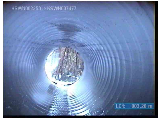
KSWP003634_23266daf-560e-4aaf-960b-442abe849b0c_20220708_155222_076.jpg, 00:01:17, 3.20m Material change / Bosspipe
