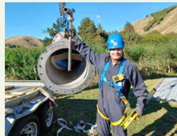
Waikanae water treatment plant upgrade.
