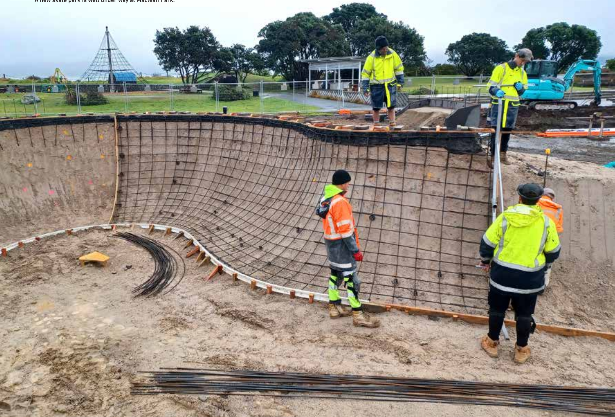
A new skate park is well under way at Maclean Park.
