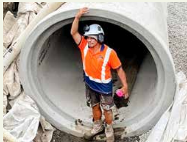
The Paraparaumu stormwater network is now completed.
