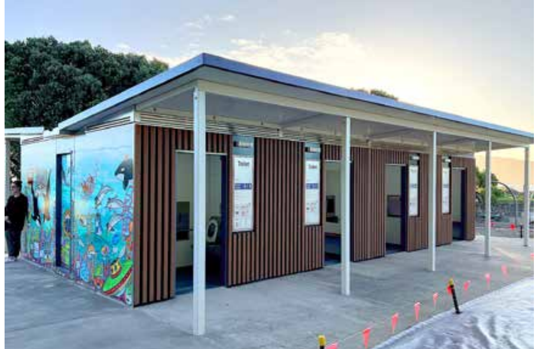
Before and after – Maclean Park amenity block.
