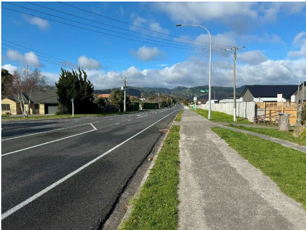
Figure 2-4: View south along Mazengarb Road (Site on the right)
