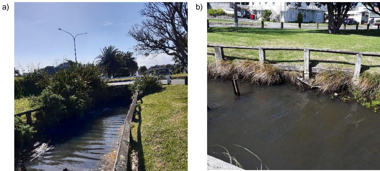
Figure 3-3 a) looking upstream, Tikotu Stream from the pedestrian bridge; b) looking from the true left (north) bank across the stream just upstream of the pedestrian bridge. .
