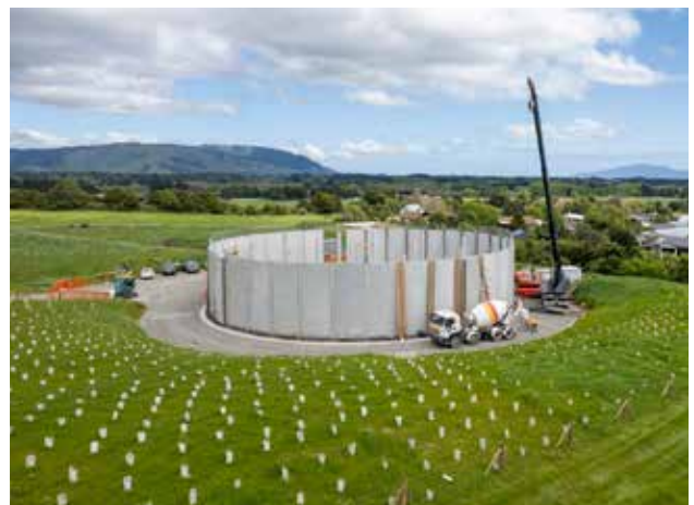
Ōtaki reservoir construction.
