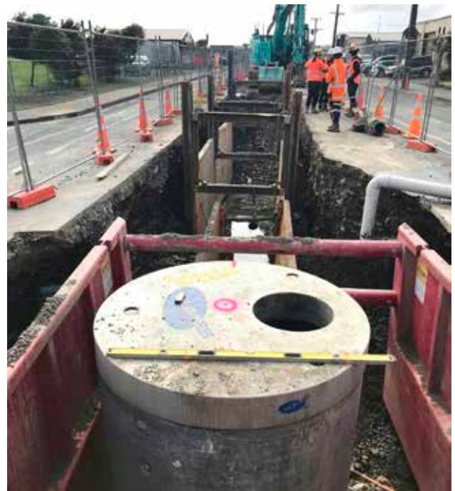
Wastewater upgrades in Ōtaki.
