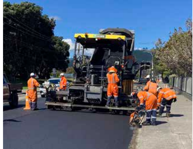
Raumati road resurfacing.
