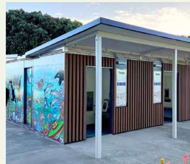
New wharepaku (toilets) and accessible changing rooms adorned with designs from a local artist were installed at Maclean Park.
