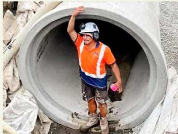
The Paraparaumu stormwater network is now completed.
