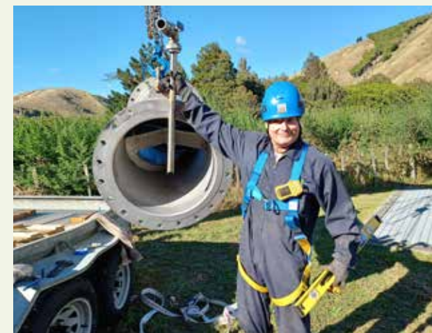
Waikanae water treatment plant upgrade.
