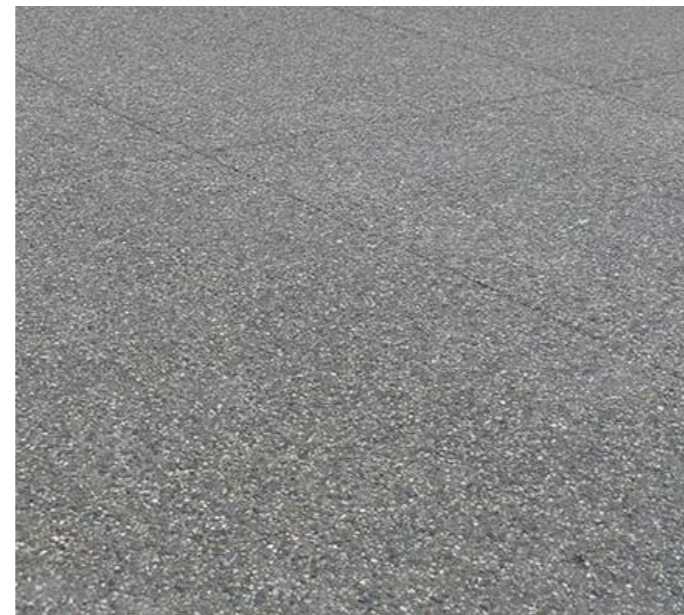
Exposed Aggregate - Driveway
