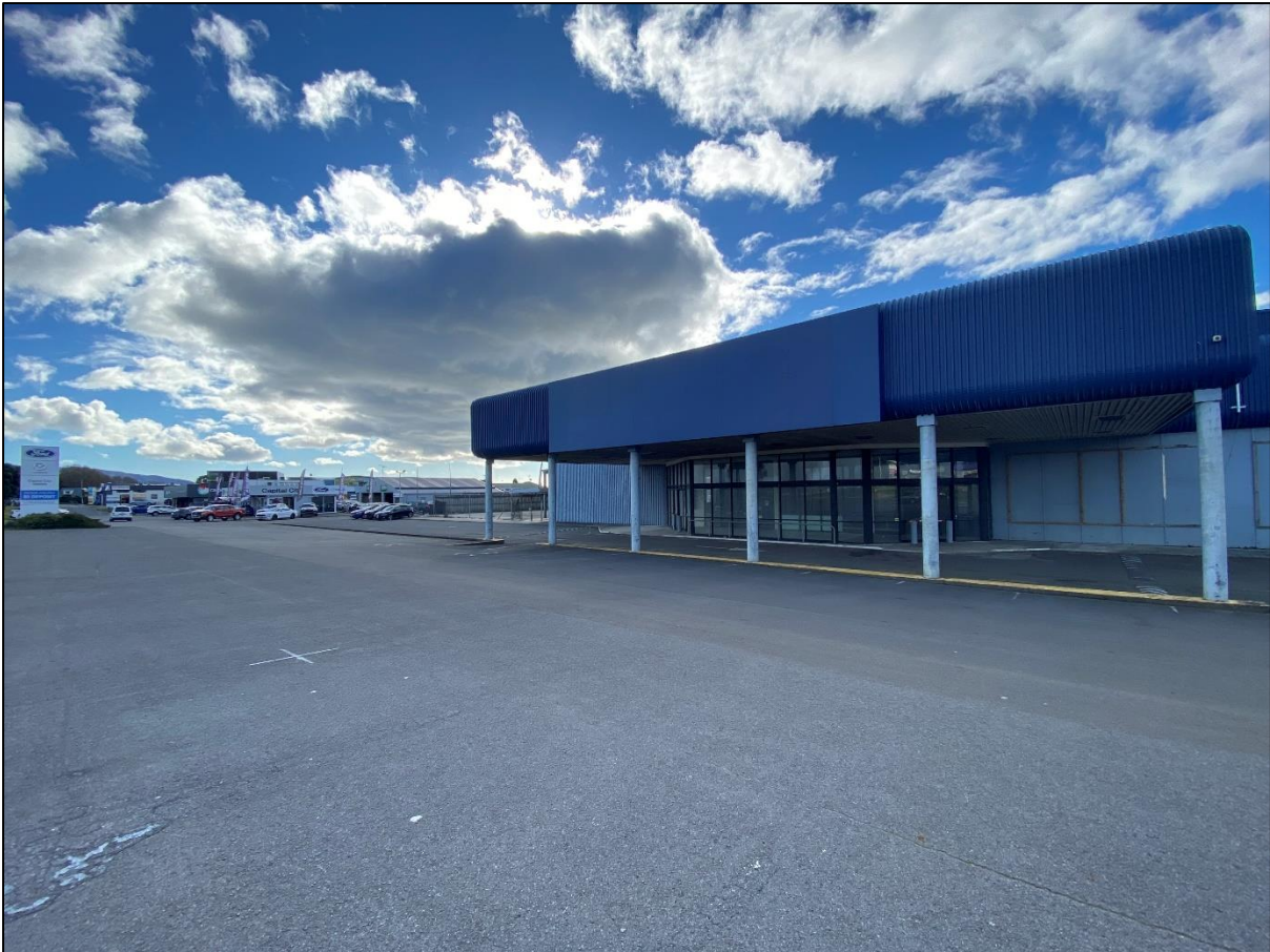
Figure 2: View from the proposed car parking of the existing building on the site to be removed
