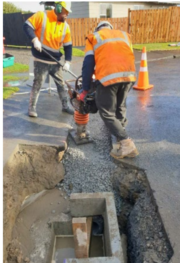
Stormwater works in central Paraparaumu.
