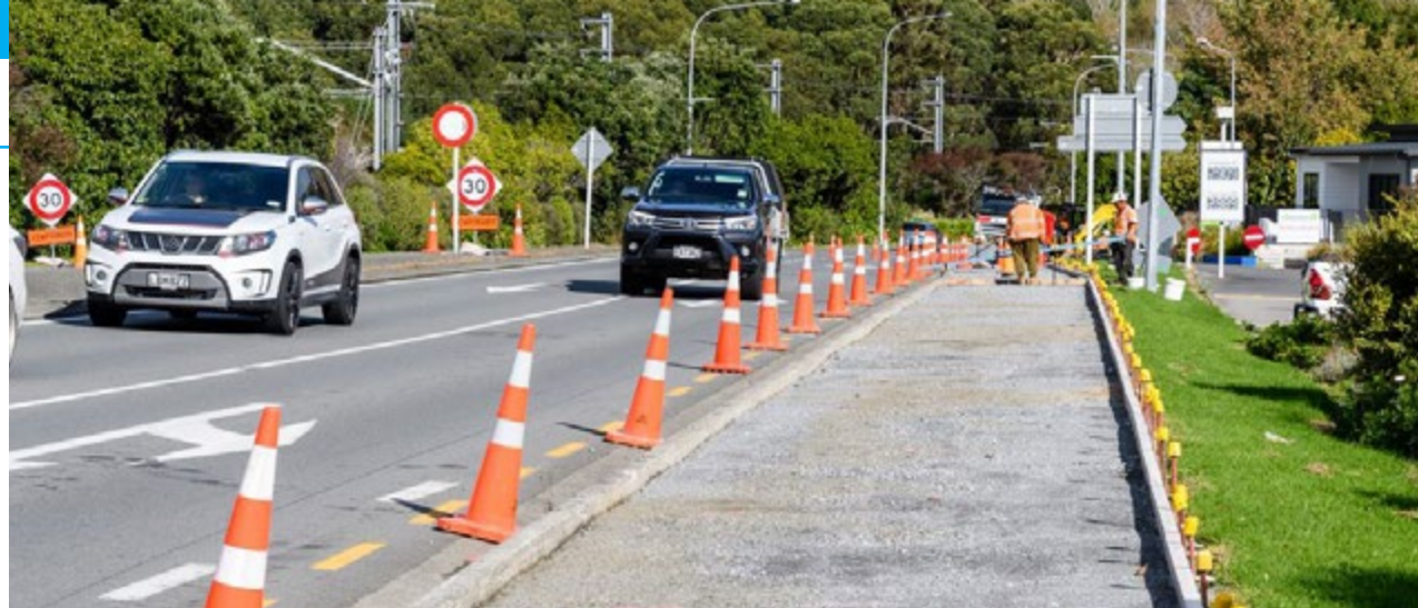
Footpath creation in Waikanae.
