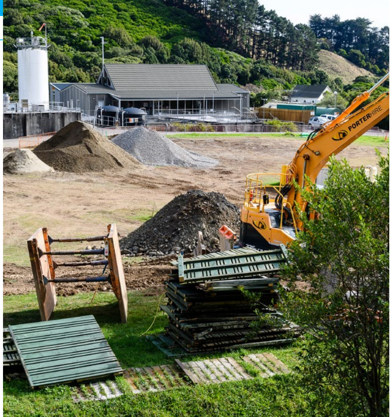
Waikanae Water Treatment Plant.
