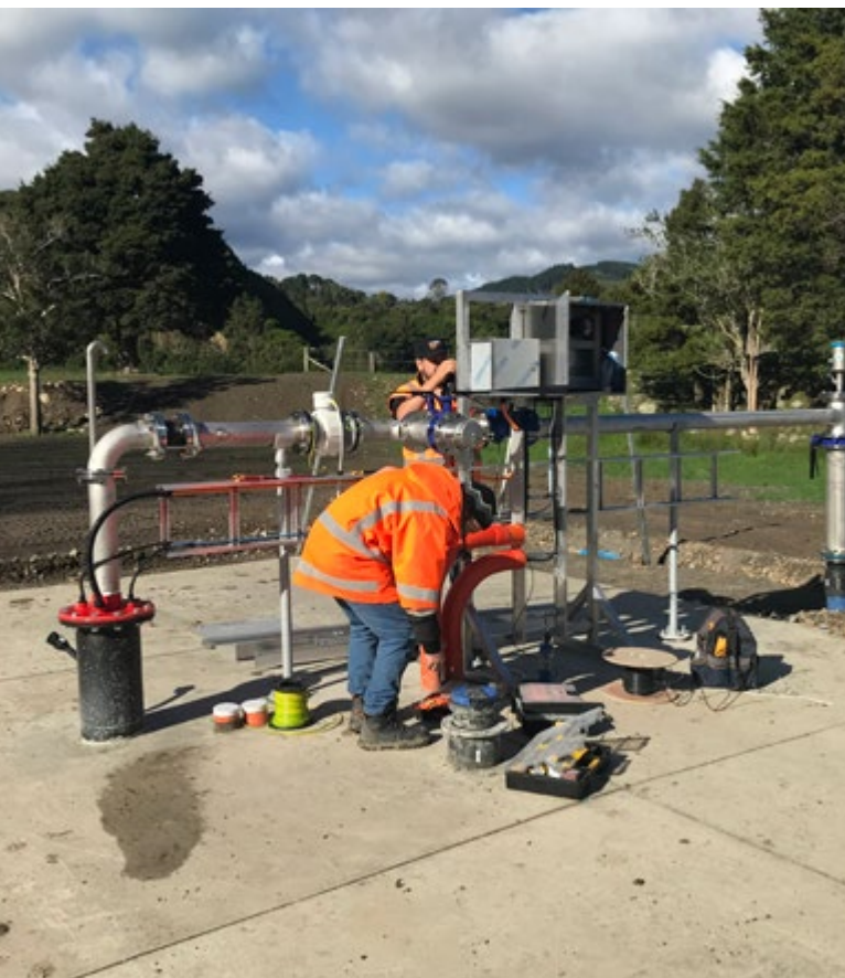
Upgrade at the Hautere water treatment plant to increase turbidity resilience.
